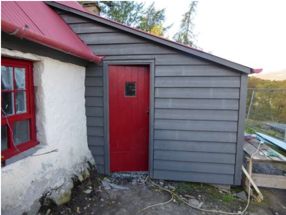
Figure 28. The rebuilt porch, on the original footings and to the same profile, which became the kitchen.
