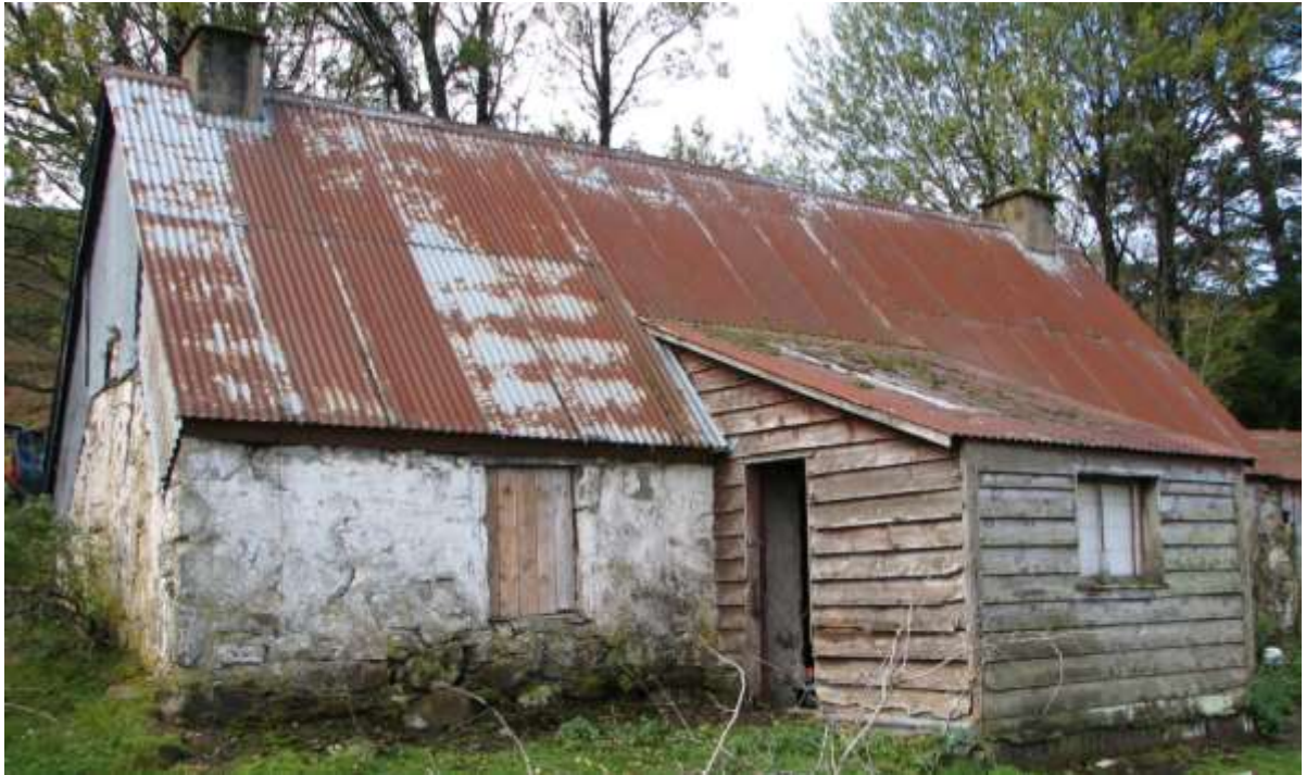
Figure 4. The Croft house in 2011 prior to the refurbishment. The corrugated iron roof covering is of relatively recent date but has largely ensured the survival of the building and the heather thatch beneath.
