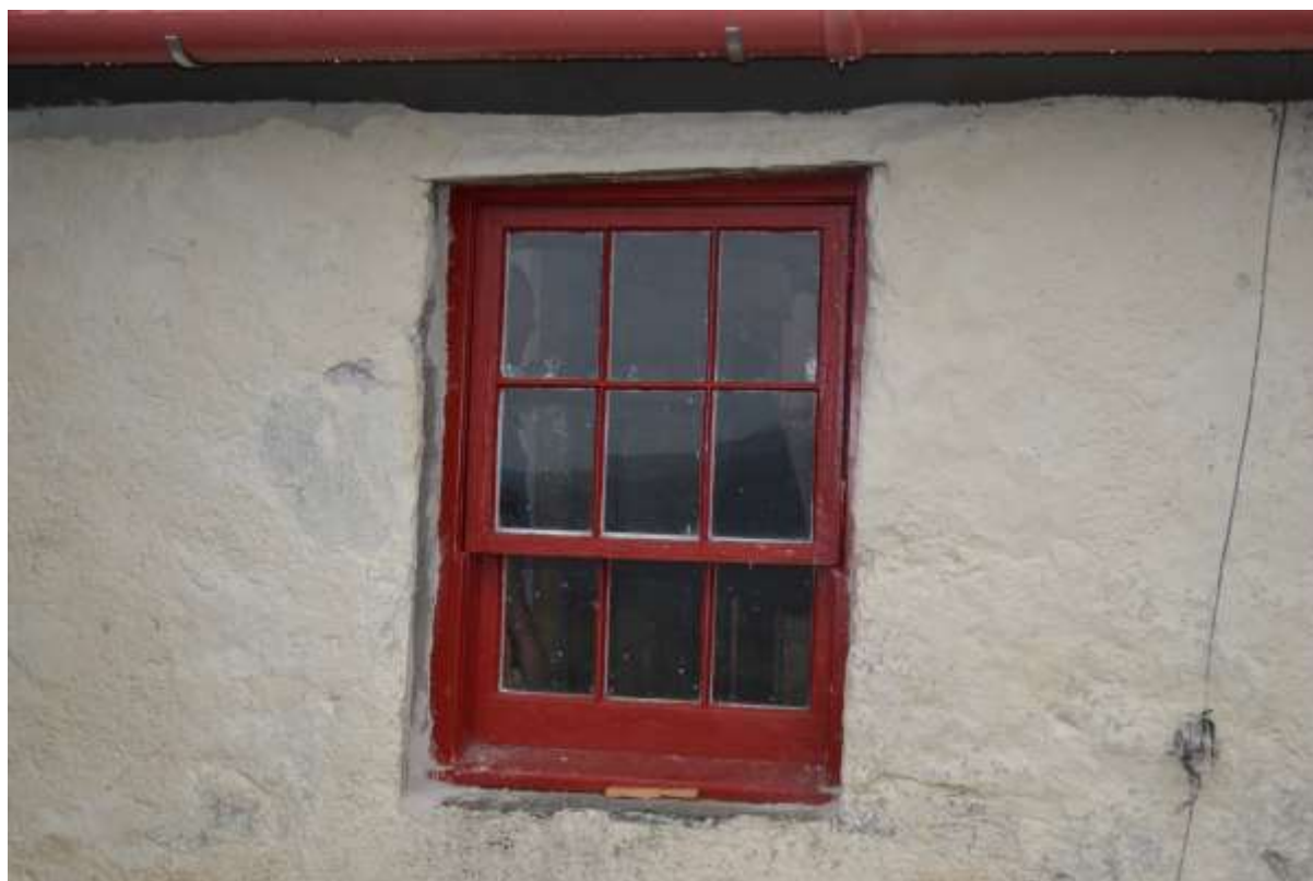
Figure 27. The repaired parlour window, following adjustment for use as a fire escape.
