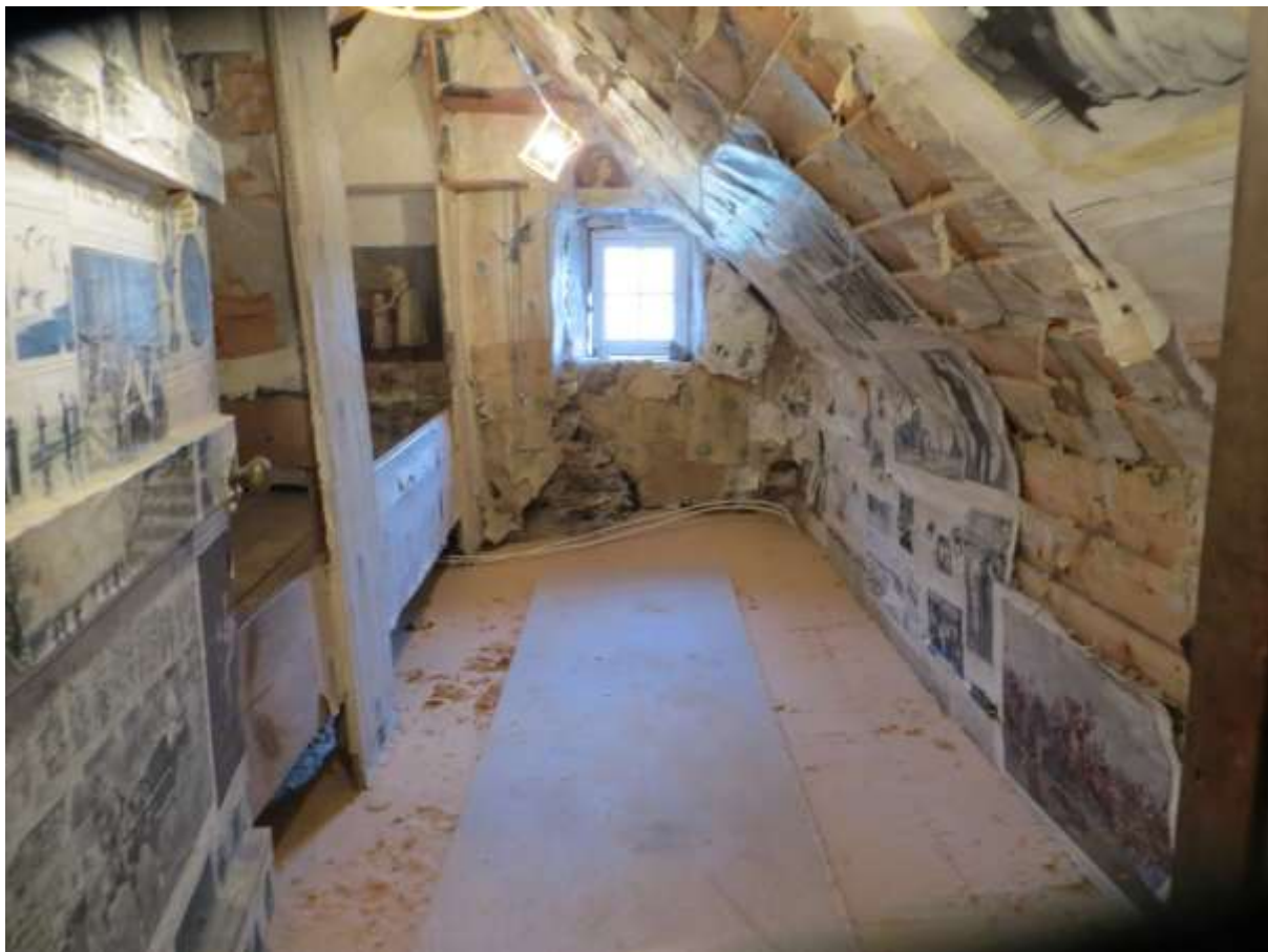
Figure 26. Wood fibre insulation laid on top of the floor in the attic rooms.
