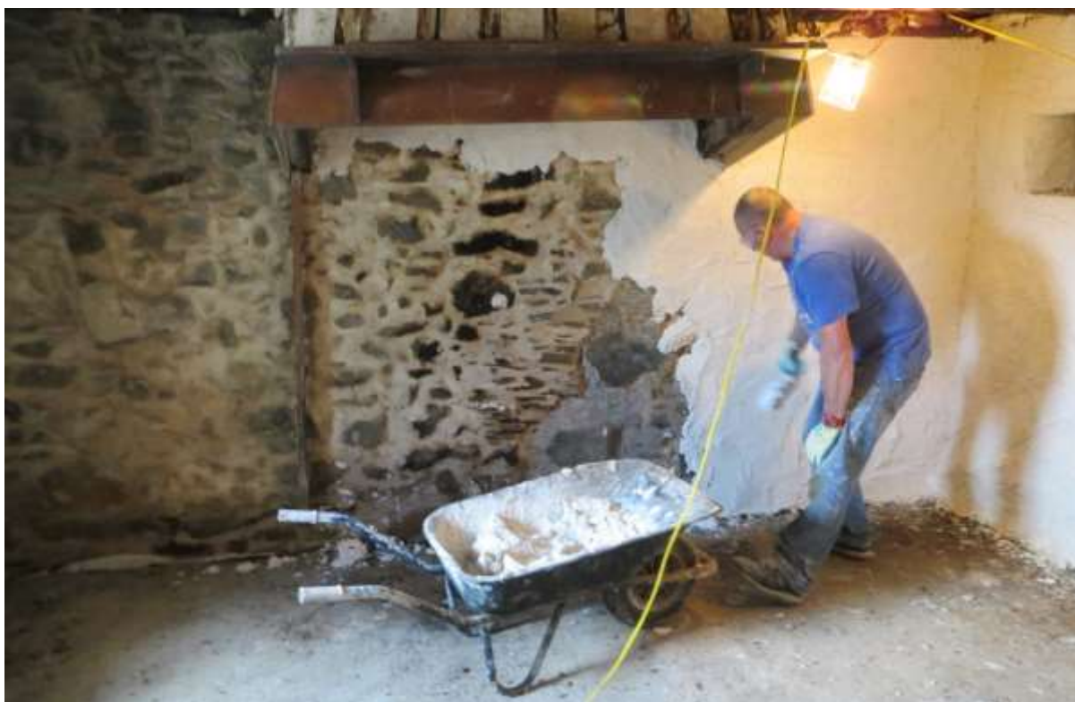
Figure 23. The first coat of insulated lime plaster being applied in the kitchen.
