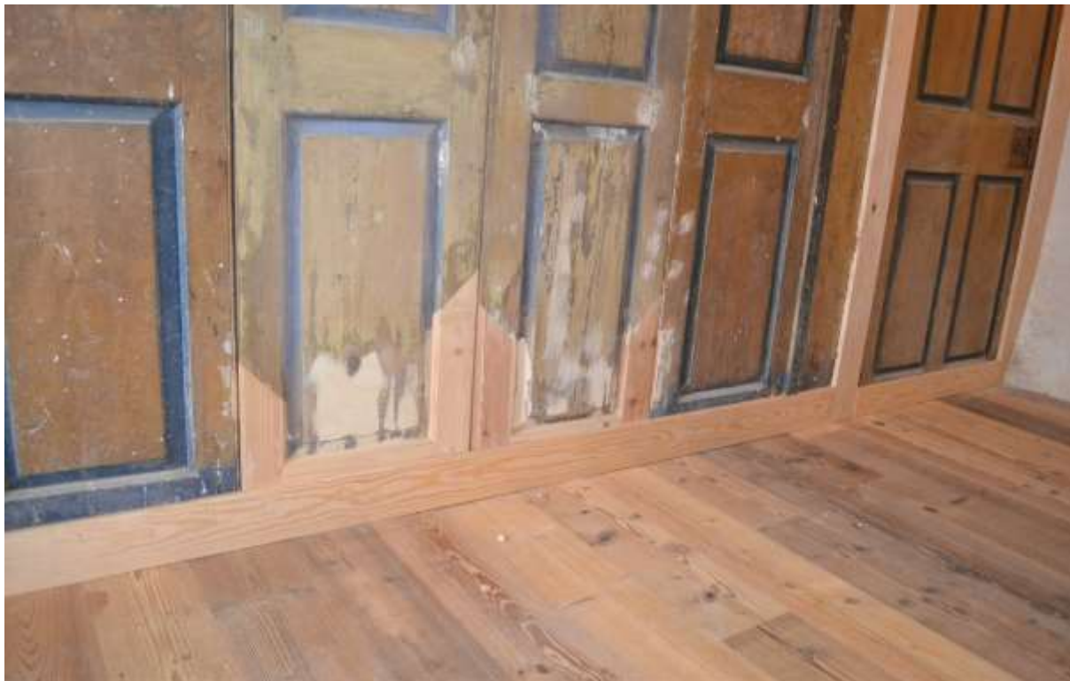
Figure 25. The new timber floor and the repaired box bed panelling in the west bedroom.
