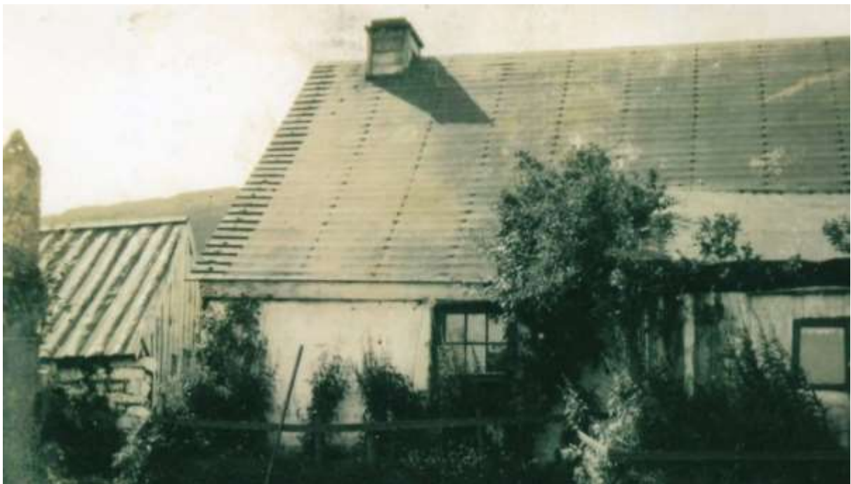
Figure 5. The croft house viewed from the north in the late 19 th century, showing the timber plank roof covering protecting the thatch. Note the steading to the left roofed with vertically laid sawn planks.
