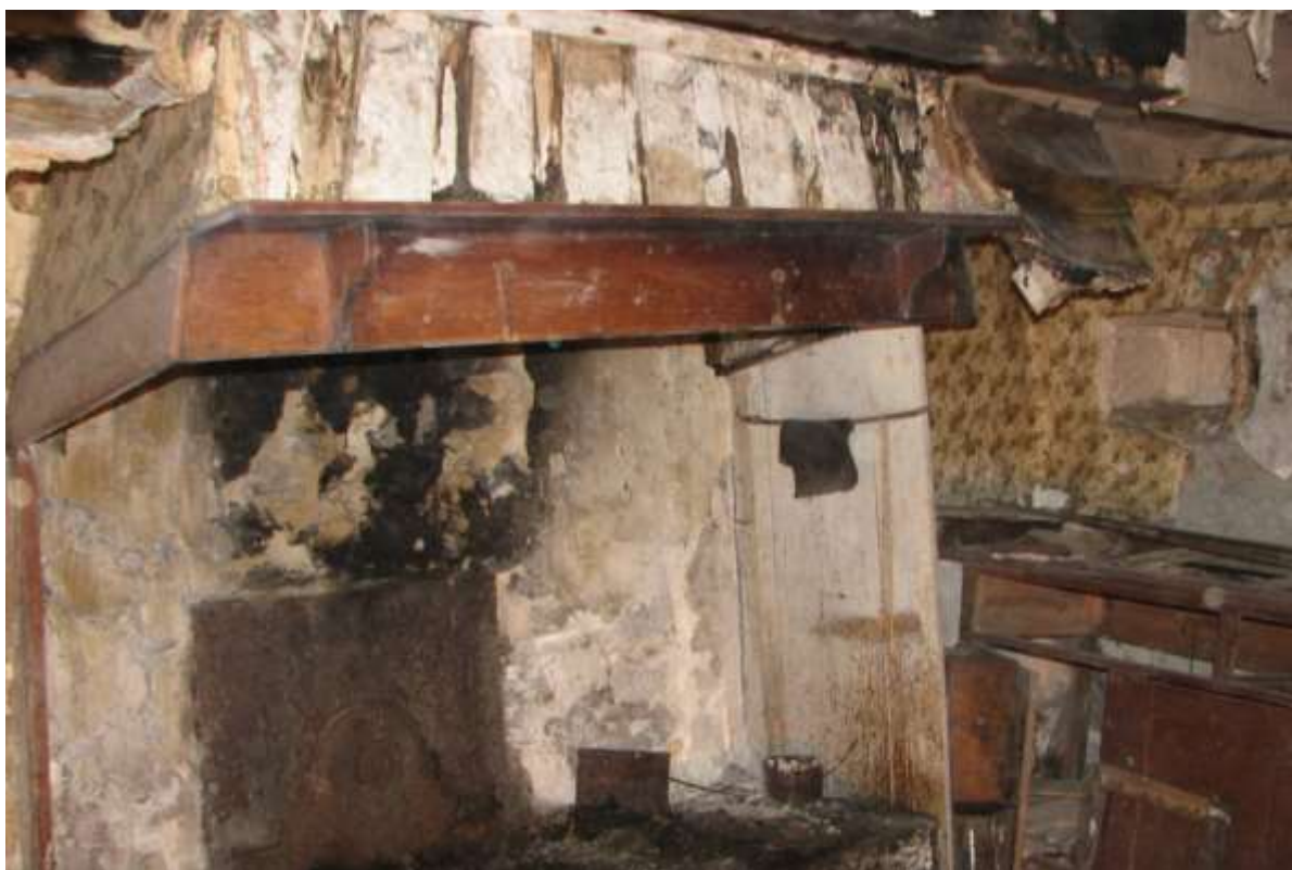
Figure 9. The hanging lum in the kitchen prior to works; a very rare survivor of a once common feature in rural homes.
