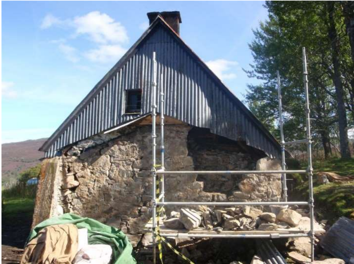
Figure 18. Rebuilding work on the west gable wall in 2013.
