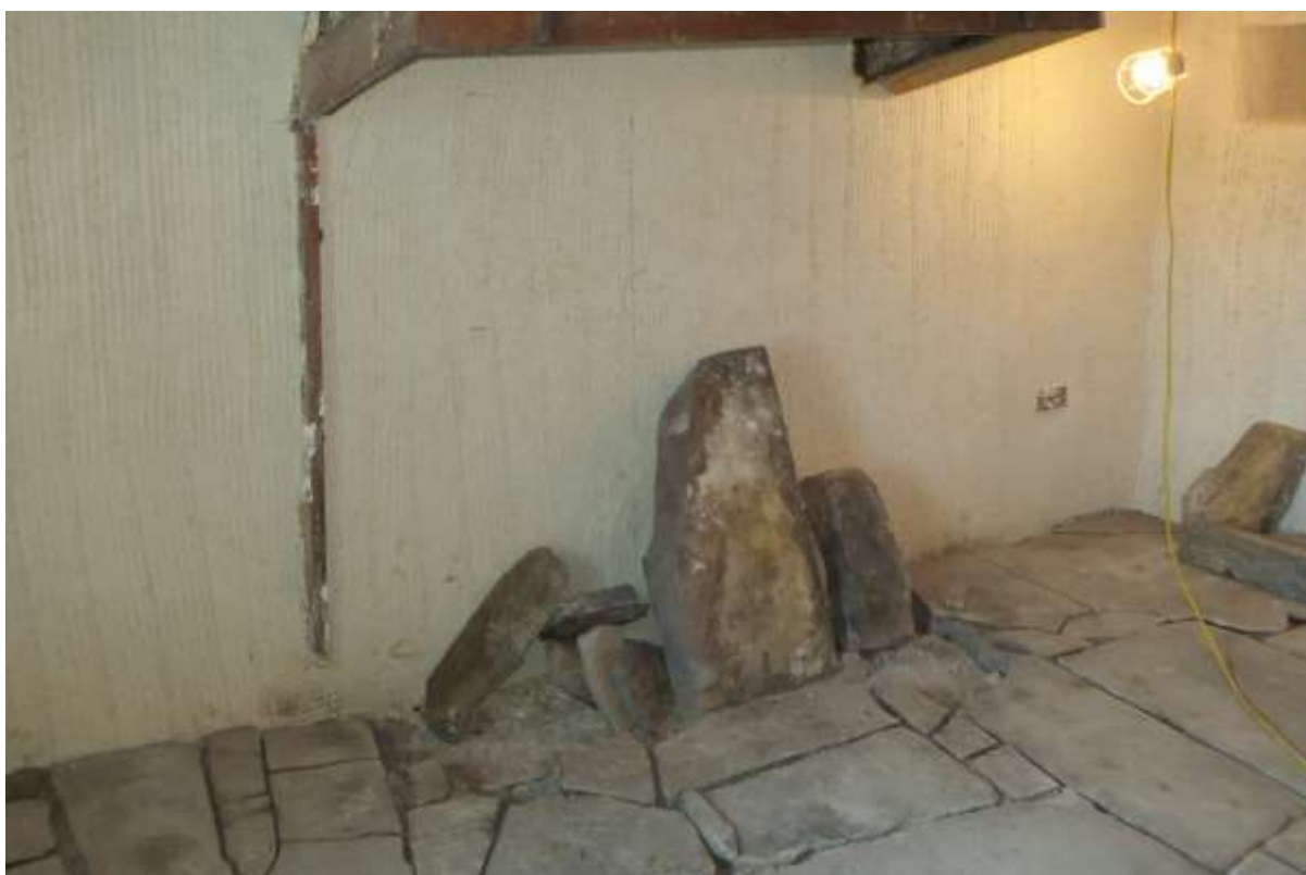
Figure 24. Re-laying the flagstones in the kitchen onto the insulated lime concrete.
