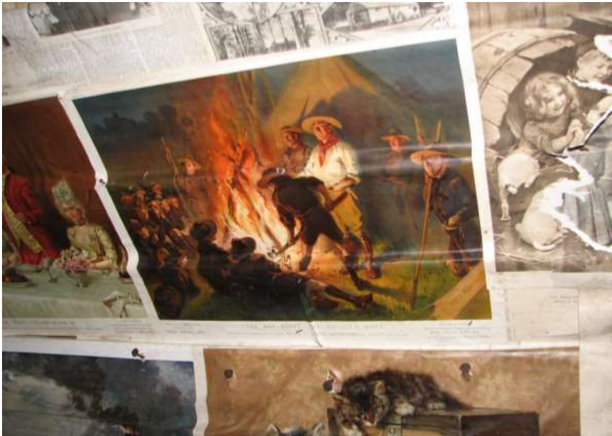
Cuttings and images from the 'Illustrated London News' used as internal wall coverings at stairwell partition
