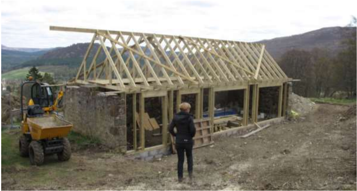
Figure 15. The new roof structure on the byre.
