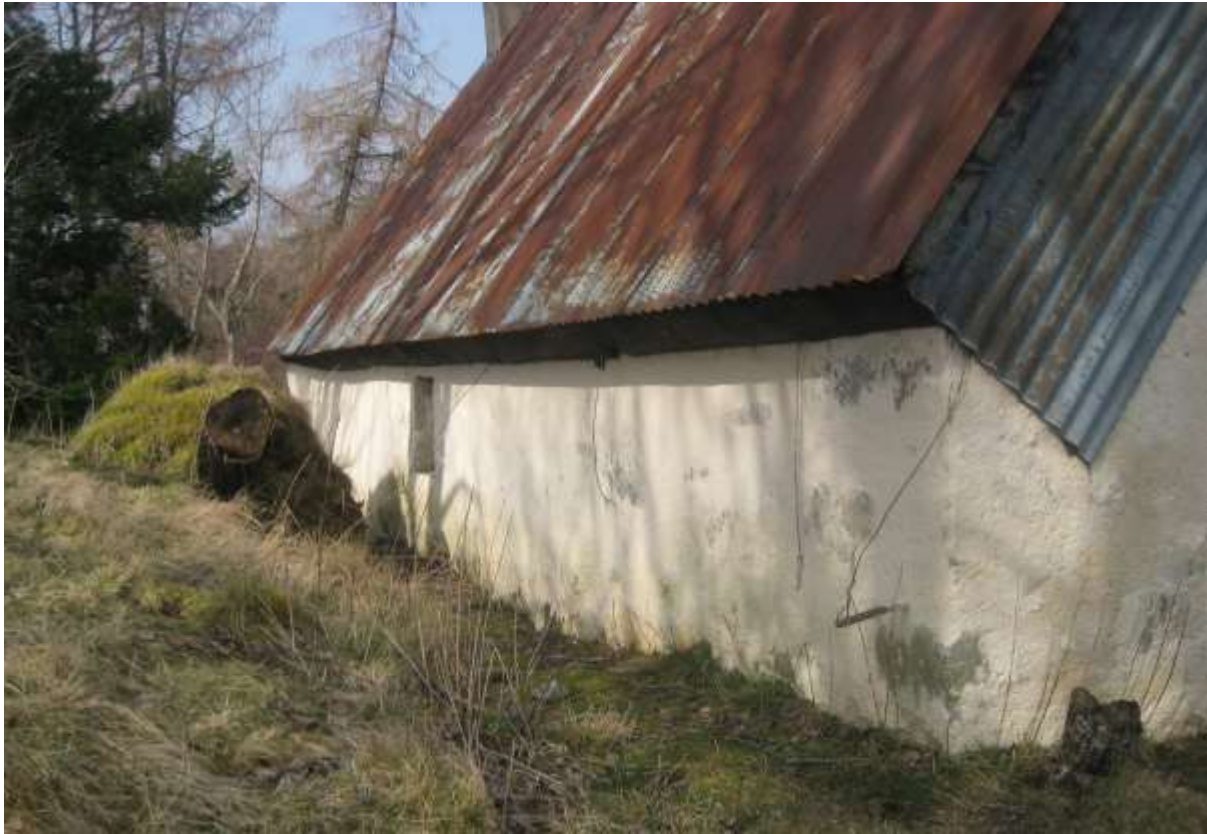
Figure 19. Completed limewash on the partly re-built south wall.
