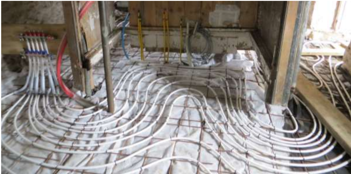
Figure 31. The heating coil fixed in place prior to the final lime concrete layer.
